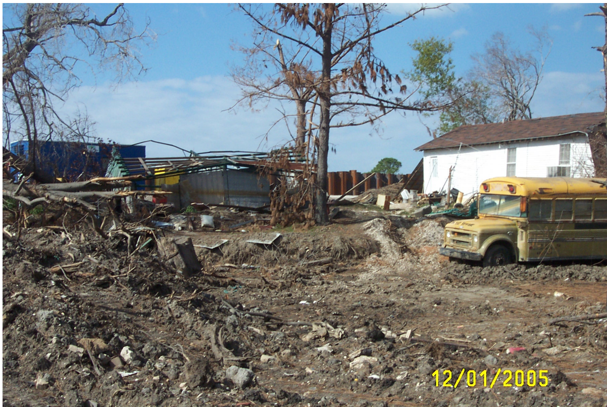
Figure 33. Slide toe (at abrupt change in slope in front of school bus) where levee and neighborhood were displaced about 45 feet toward the viewer.
