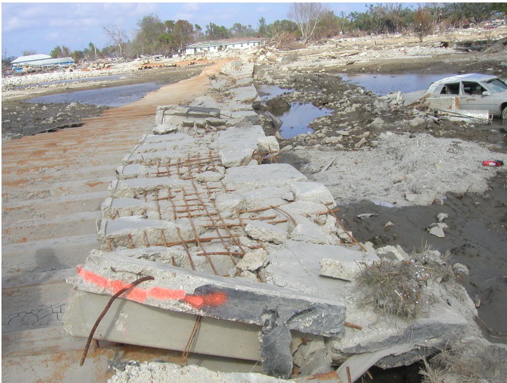
Figure 12. Floodwall and sheet piling strewn into Lower 9 th Ward at the southern (larger) breach on the Industrial Canal. Photo from U.S. Army Corps of Engineers IPET web site, taken October 4, 2005.
