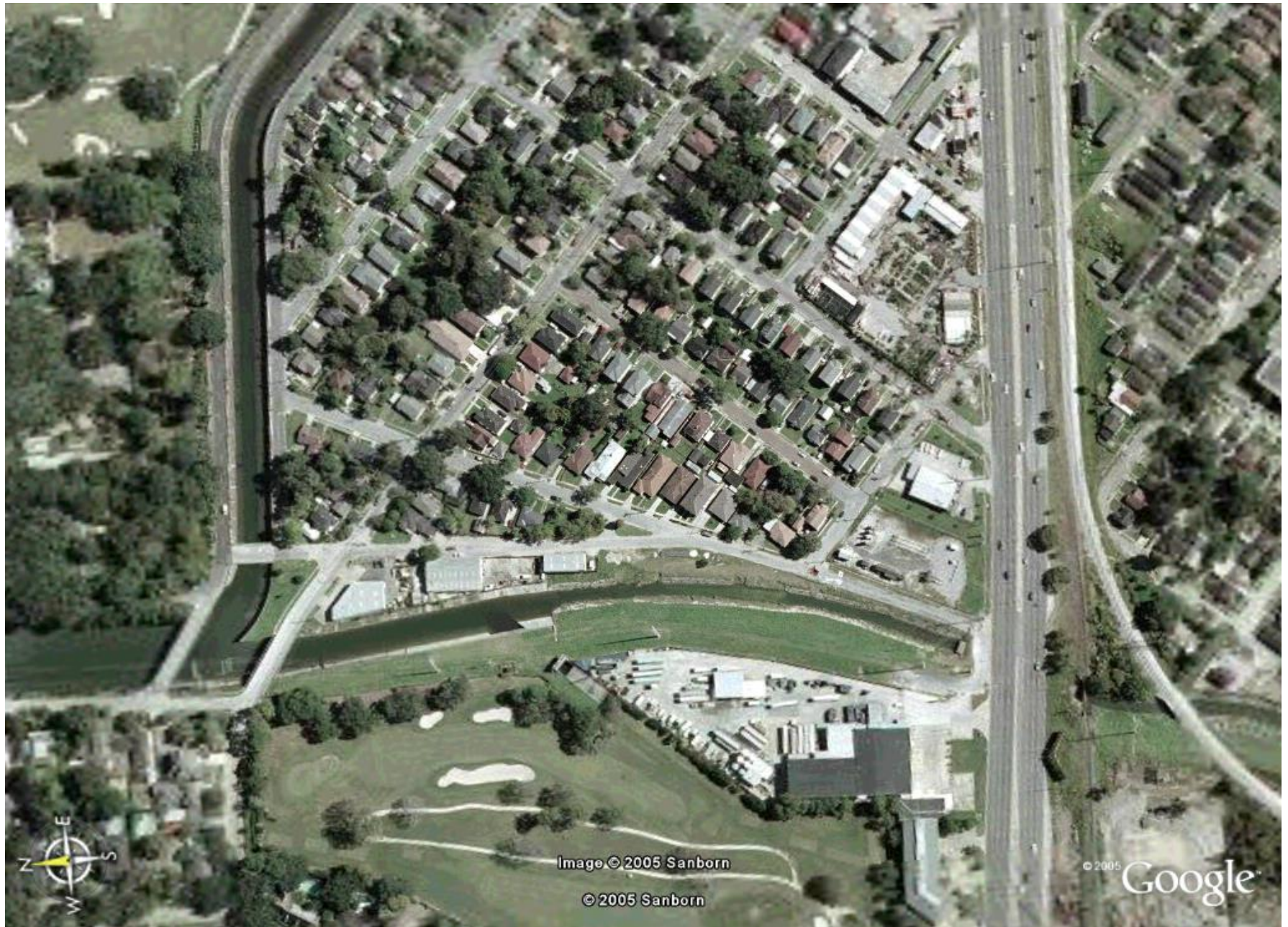
Figure 42. Satellite image of the area near the southern end of the 17th Street Canal near Old Metairie where water would enter Jefferson Parish from levee breaches in Orleans Parish during Hurricane Katrina (Stop 7). (Source - Google Earth)
