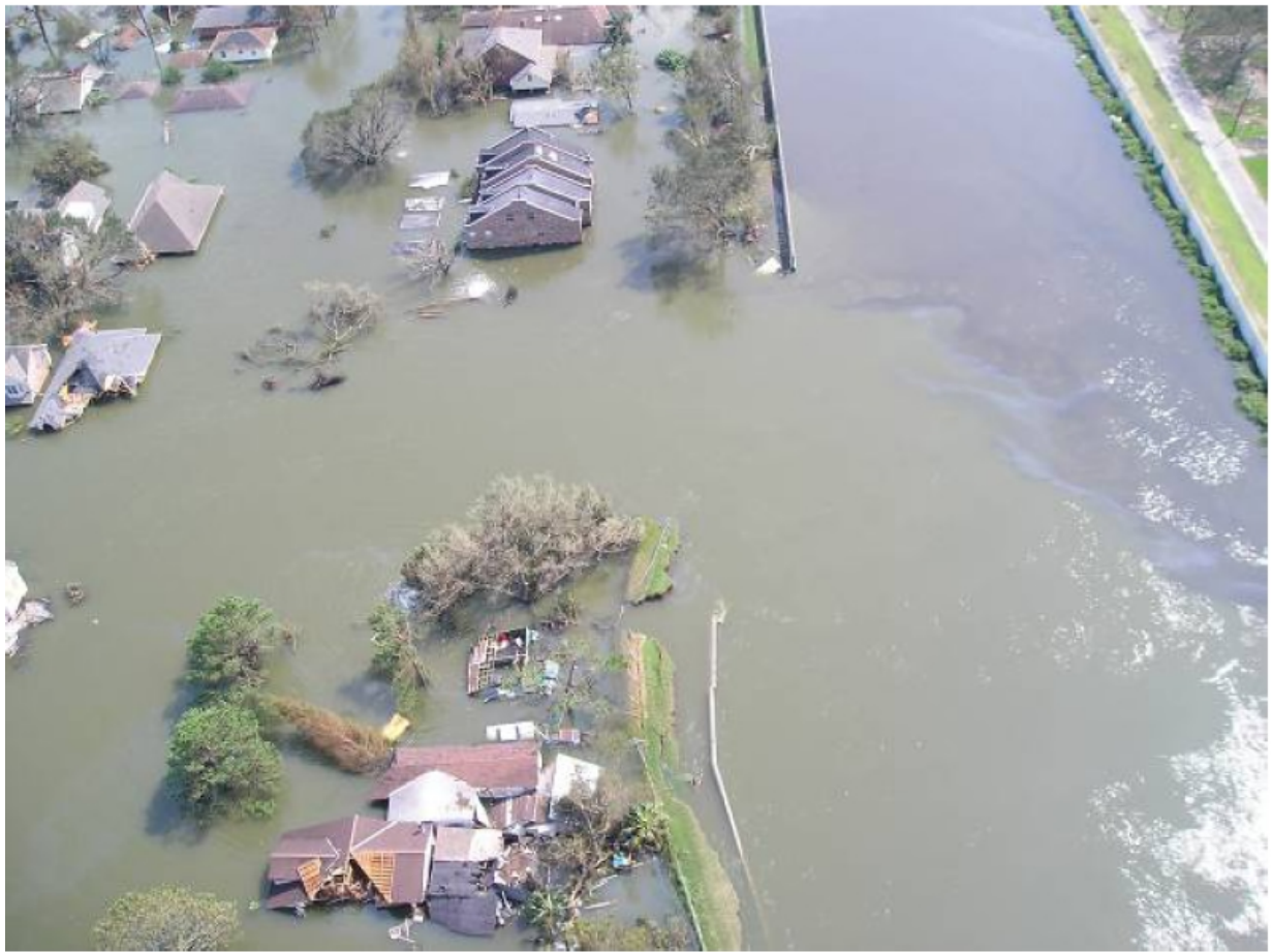
Figure 31. View of 17 th St. Canal breach looking toward south. Note displaced floodwall and levee just below the missing section of the levee.
