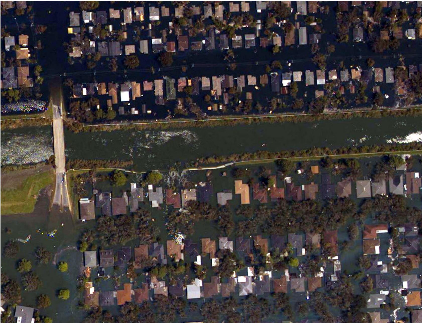
Figure 25. Air photograph of the area where the London Avenue Canal levee was breached near Robert E. Lee Ave. and Pratt Drive (Stop 2). Drive. Image acquired Aug. 31, 2005. Source: National Oceanic and Atmospheric Administration's National Geodetic Survey, Katrina Images - http://ngs.woc.noaa.gov/katrina/
