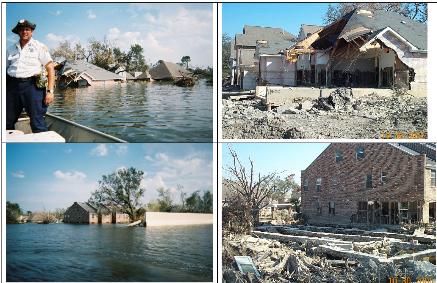
Figure 38. Comparison of water levels on Sept.1, 2005 (photos on left by Kevin Himmel), with water lines on same structures indicate lines left by standing water are about 1.5 to 2 feet lower than the maximum water level. Note large block of peat in photo at the upper right. In photo at lower right, note the chainwall foundation of a house that was removed by the burst of water when the levee was breached and the cypress stump from a tree that was probably cut down 100 years ago when this Lakeview neighborhood was reclaimed from the cypress swamp.
