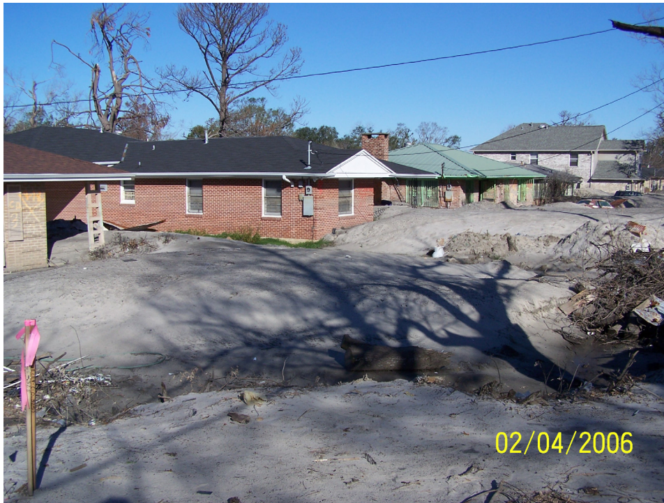
Figure 22. Sand deposits on Warrington drive showing deposition in the wake of houses as the currents flowed down the driveways between the houses. As of March 1, 2006, most of the sands deposits have been removed.
