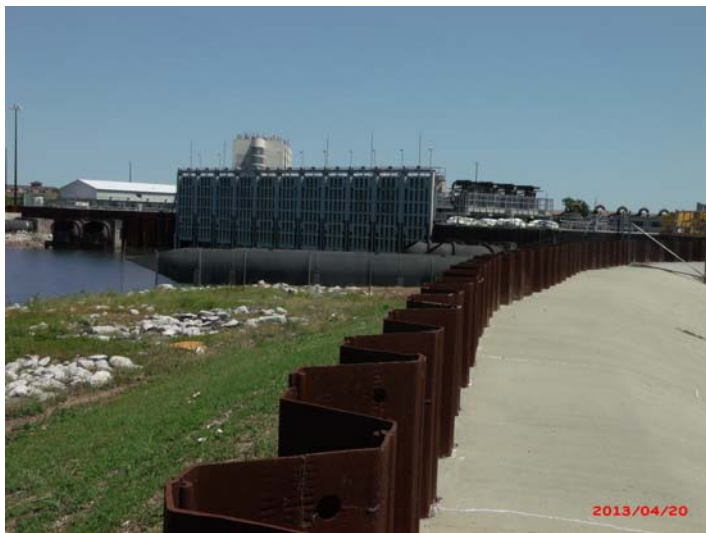
Figure 41. Gate and pumps near the Lake end of the London Avenue Canal (Stop 6).
