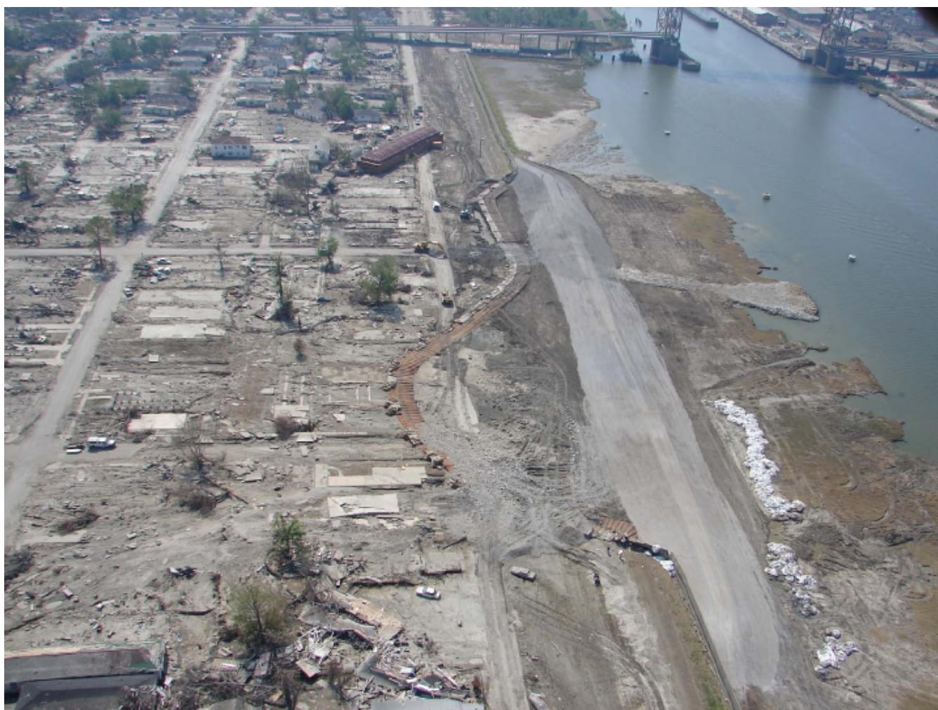
Figure 14. View of southern breach on the Industrial Canal, looking South. Note the floodwall and sheet piling (brown) strewn through the Lower Ninth Ward neighborhood where all houses were removed by the force of water coming through the breach. Gray deposits on right are breach repair gravels. Note barge near in the center near the top of the photo. Photo by L. Harder - Independent Levee Investigation Team Final Report (2006).
