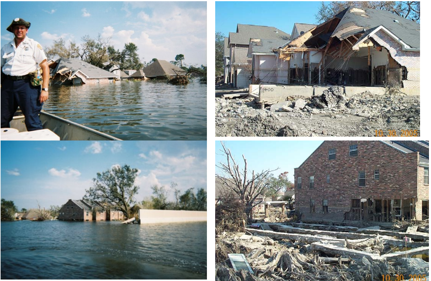
Figure 51. Comparison of water levels on Sept.1, 2005 (photos on left by Kevin Himmel), with water lines on same structures indicate lines left by standing water are about 1.5 to 2 feet lower than the maximum water level. Note large block of peat in photo at the upper right. In photo at lower right, note the chainwall foundation of a house that was removed by the burst of water when the levee was breached and the cypress stump from a tree that was probably cut down 100 years ago when this Lakeview neighborhood was reclaimed from the cypress swamp.
