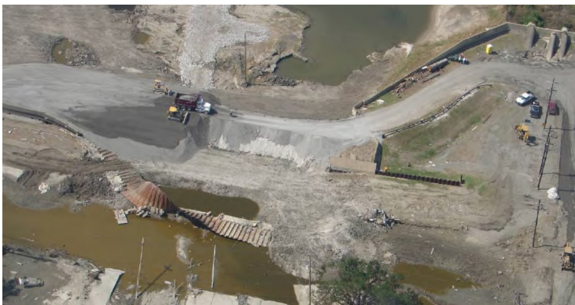
Figure 16. Aerial view of the north breach on Industrial Canal. Photo by L. Harder - Independent Levee Investigation Team Final Report (2006).
