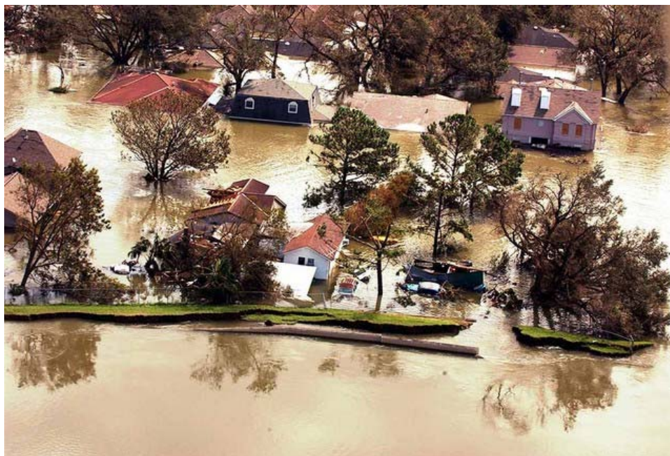
Figure 44. View of 17 th St. Canal breach looking toward east. Note fractures in the displaced part of the levee. Photo by J. Augustino FEMA.
