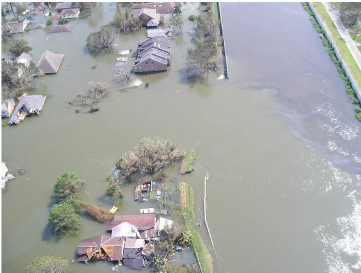
Figure 43. View of 17 th St. Canal breach looking toward south. Note displaced floodwall and levee just below the missing section of the levee. Photo from IPET Report .
