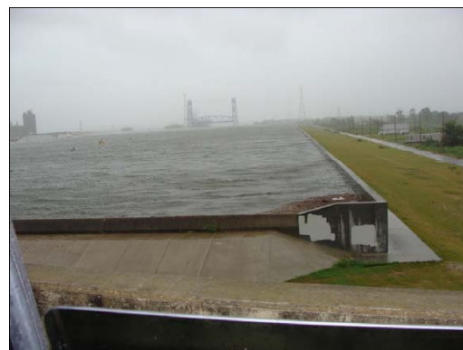
Figure 23. View of the Industrial Canal from the Claiborne Ave. Bridge looking North toward Stop 7 with the Florida Ave. Bridge (blue bridge) on the horizon. Photo as taken on the morning of Sept. 1, 2008 during the passage of Hurricane Gustav. Note the elevation drop from the post-Katrina floodwall (on the right) to the original floodwall to the left. Photo from U.S. Army Corps of Engineers.
