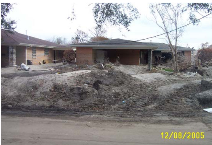
Figure 40. Sand deposits in front of houses on Pratt Drive at the North breach of the London Ave. Canal.
