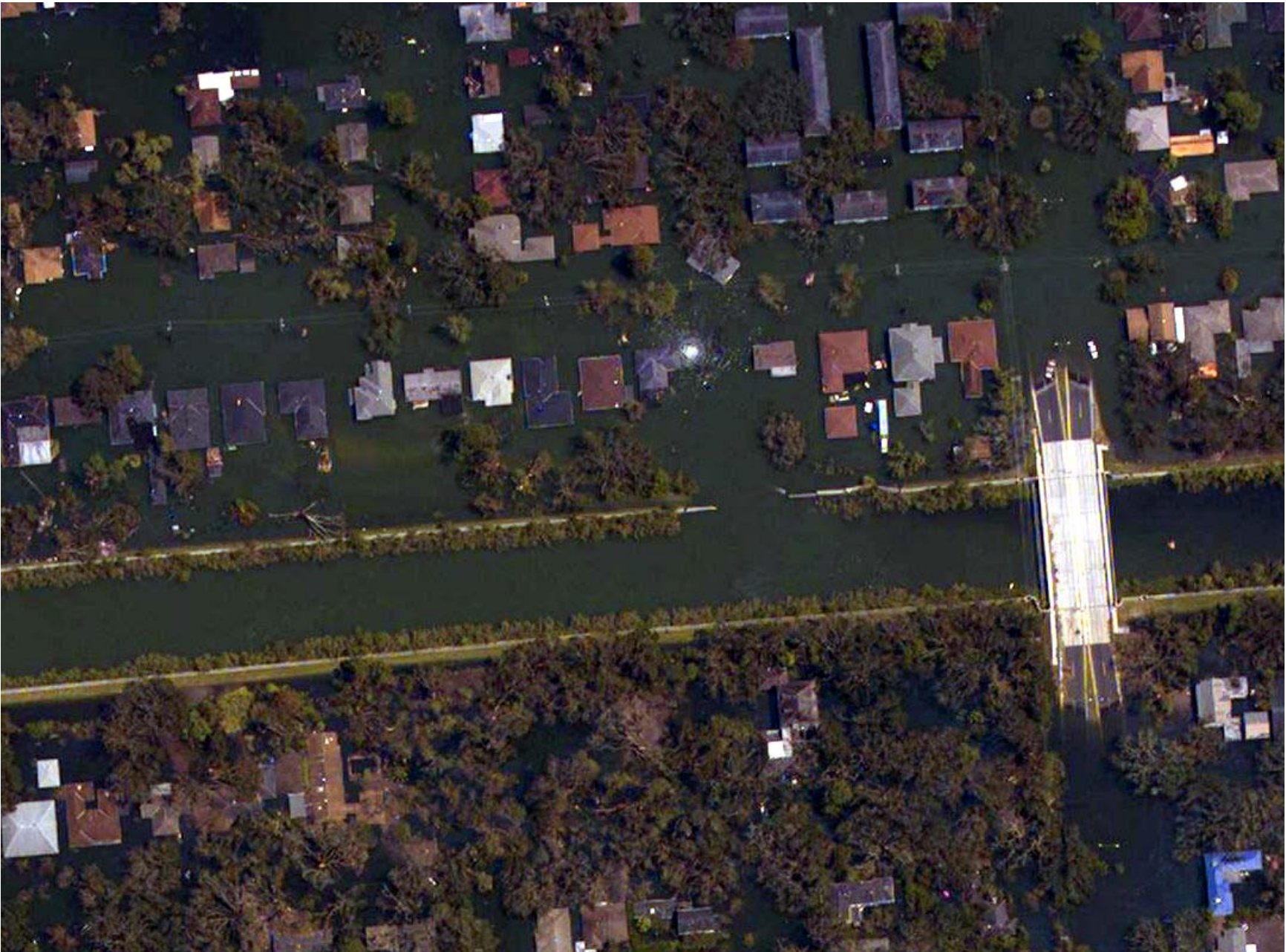
Figure 28. Air photograph of the area where the London Avenue Canal levee was breached near Mirabeau Ave. and Warrington Drive (Stop 4). Image acquired Aug. 31, 2005. Source: National Oceanic and Atmospheric Administration's National Geodetic Survey, Katrina Images - http://ngs.woc.noaa.gov/katrina/
