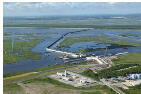
Figure 24. The surge barrier and navigation gates across the Intracoastal Waterway and MR-GO (see location in Figure 1), designed to prevent storm surge from entering the Industrial Canal.
