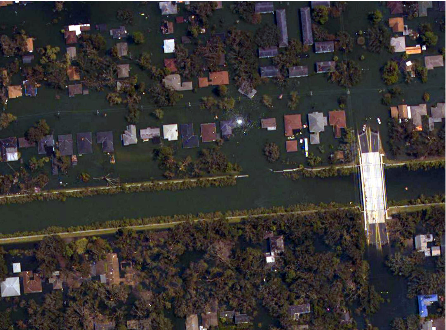
Figure 25. Air photograph of the area where the London Avenue Canal levee was breached near Mirabeau Ave. and Warrington Drive (Stop 2). Image acquired Aug. 31, 2005. Source: National Oceanic and Atmospheric Administration's National Geodetic Survey, Katrina Images - http://ngs.woc.noaa.gov/katrina/
