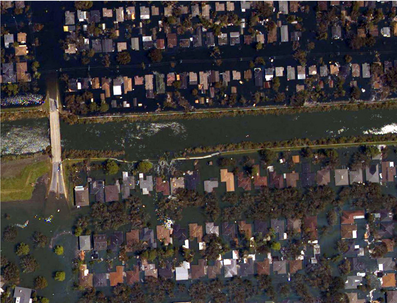
Figure 32. Air photograph of the area where the London Avenue Canal levee was breached near Robert E. Lee Ave. and Pratt Drive (Stop 3). Drive. Image acquired Aug. 31, 2005. Source: National Oceanic and Atmospheric Administration's National Geodetic Survey, Katrina Images - http://ngs.woc.noaa.gov/katrina/
