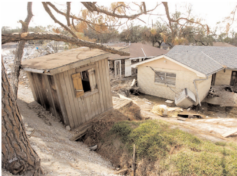
Figure 34. Child's clubhouse behind the Cantrell home on Pratt Drive uplifted along the west side of the London Avenue Canal near the breach (Stop 3). Note the fractures beneath and in front of (right side in photo) the clubhouse. Gray material at base of tree is gravel used in the repair of the breach. Source: Times-Picayune Tuesday, October 4, 2005. See reference to article by John McQuaid, same date
