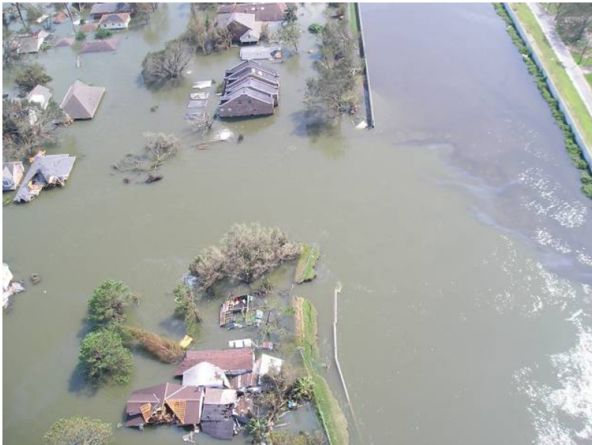
Figure 40. View of 17 th St. Canal breach looking toward south. Note displaced floodwall and levee just below the missing section of the levee. Photo from IPET Interim Report 2.
