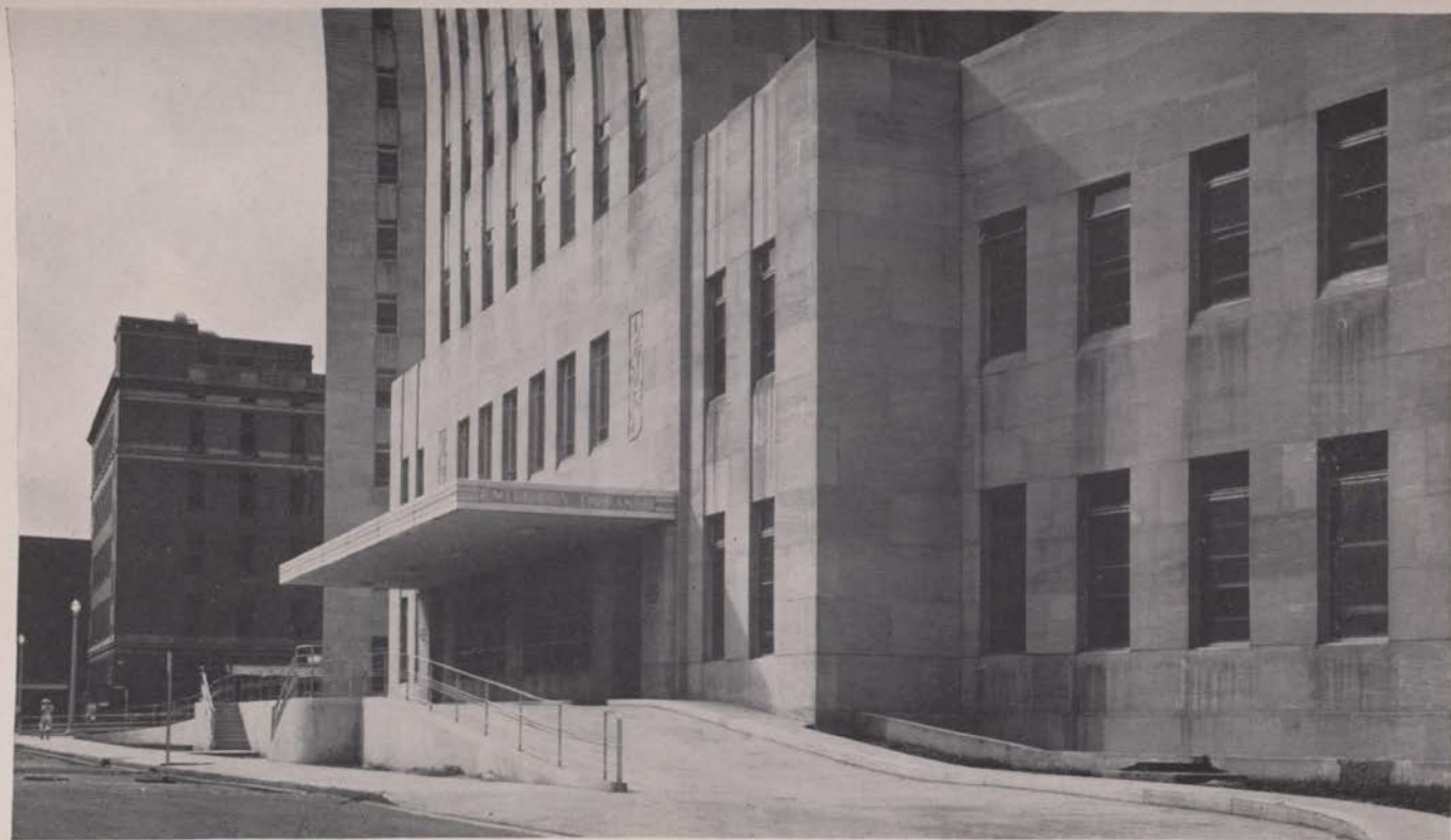
Emergency Entrance Showing Ramp for Ambulances.
