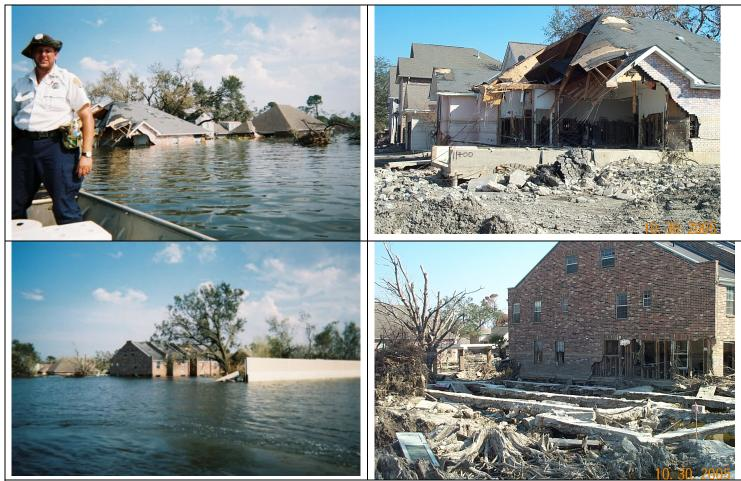
**Figure 31.** Comparison of water levels on Sept.1, 2005 (photos on left by Kevin Himmel), with water lines on same structures indicate lines left by standing water are about 1.5 to 2 feet lower than the maximum water level.
