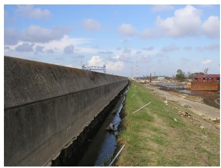
**Figure 11.** Looking North along the floodwall of the Industrial Canal levee showing trenches eroded by water from the Industrial Canal that overtopped the floodwall. Photo from U.S. Army Corps of Engineers IPET web site, taken October 4, 2005.
