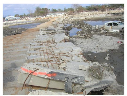
**Figure 12.** Floodwall and sheet piling strewn into Lower 9<sup>th</sup> Ward at the southern (larger) breach on the Industrial Canal. Photo from U.S. Army Corps of Engineers IPET web site, taken October 4, 2005.
