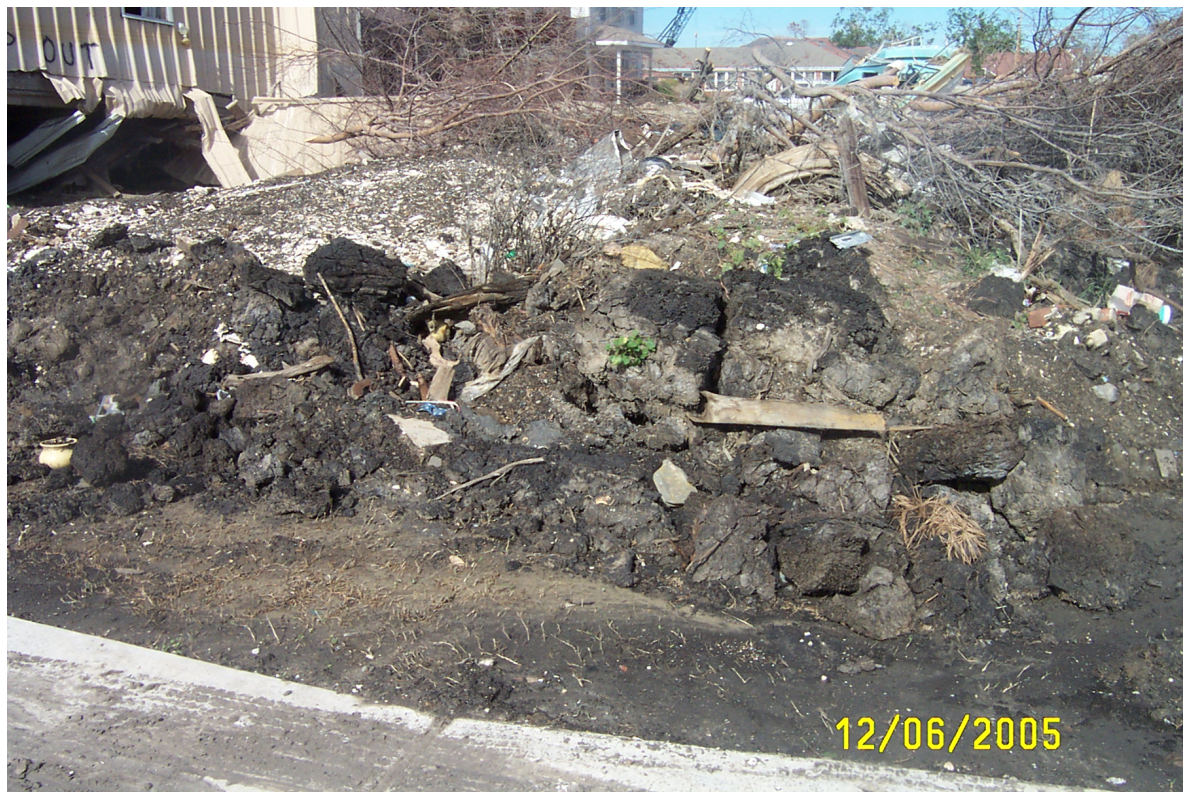
Figure 34. Blocks of Peat along Belaire Drive near the 17 th St. Canal levee breach
