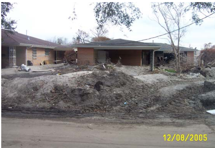
Figure 40. Sand deposits in front of houses on Pratt Drive at the North breach of the London Ave. Canal.
