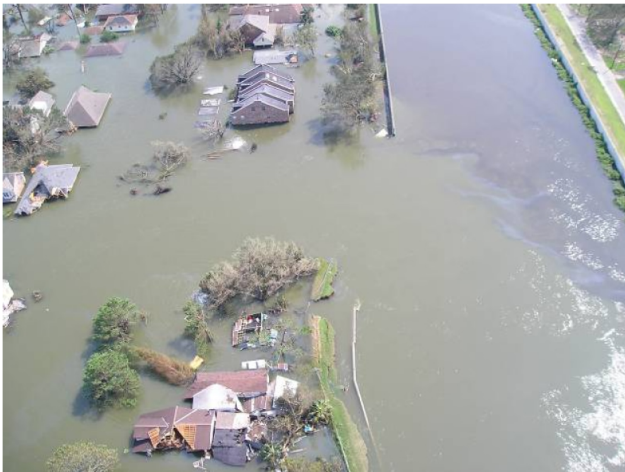
Figure 43. View of 17 th St. Canal breach looking toward south. Note displaced floodwall and levee just below the missing section of the levee. Photo from IPET Report .
