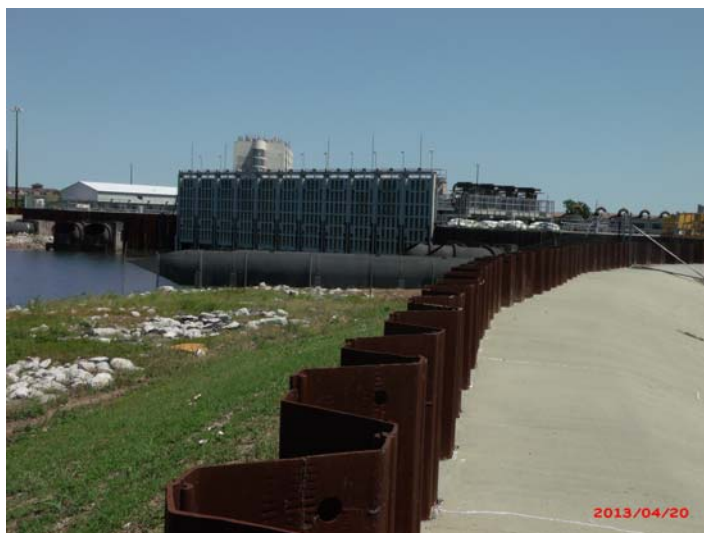
Figure 41. Gate and pumps near the Lake end of the London Avenue Canal (Stop 6).
