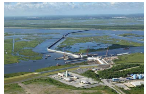
Figure 24. The surge barrier and navigation gates across the Intracoastal Waterway and MR-GO (see location in Figure 1), designed to prevent storm surge from entering the Industrial Canal.
