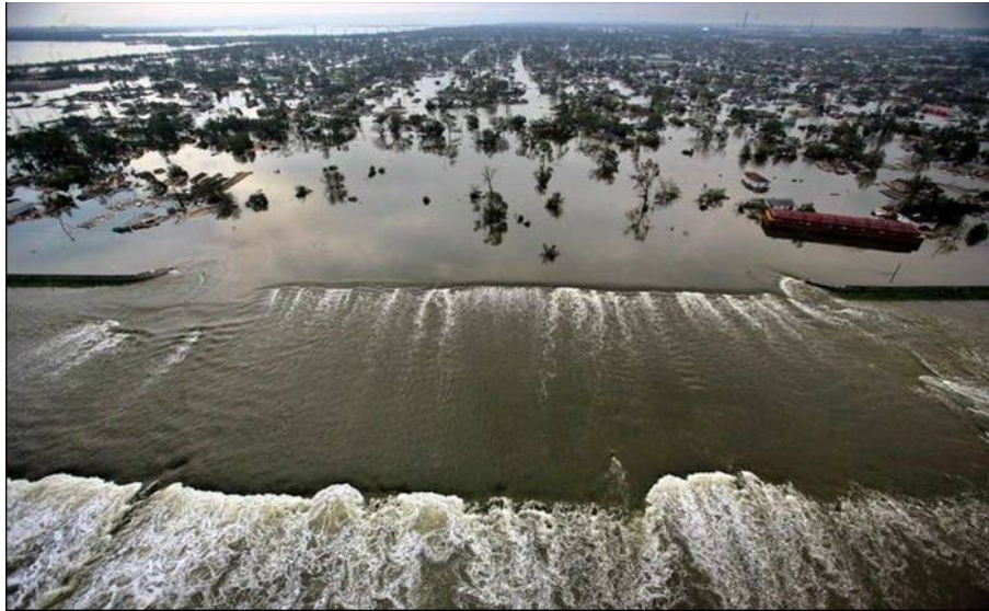
Figure 13. The large breach in the Industrial canal that flooded the Lower Ninth Ward could have been caused by a barge crashing through the floodwall during Katrina. Alternatively the barge could have floated in after the levee and floodwall were breached. Note the barge in the photo above. Note also that at the time of this photo water was running out of the Lower Ninth Ward back into the Industrial Canal. (Source - Vincent Laforet, AFP/Getty Images)
