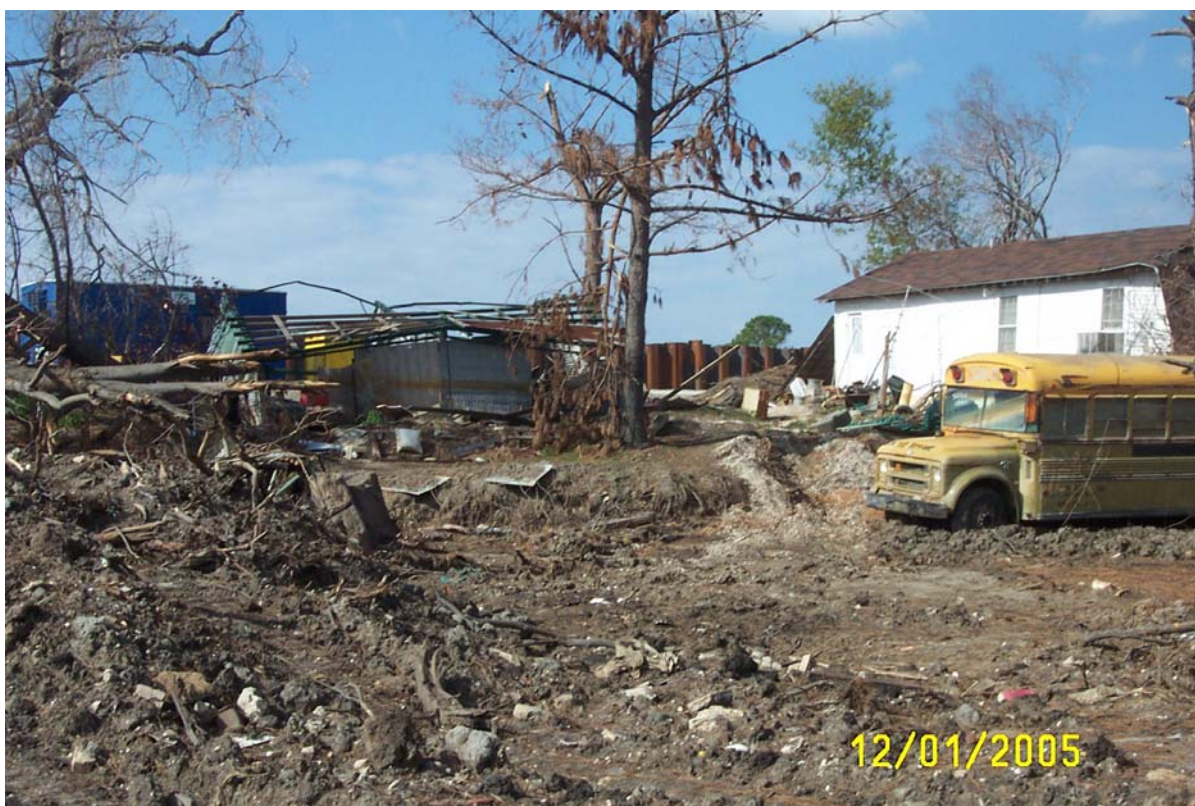
Figure 45. . Slide toe (at abrupt change in slope in front of school bus) where levee and neighborhood were displaced about 45 feet toward the viewer.
