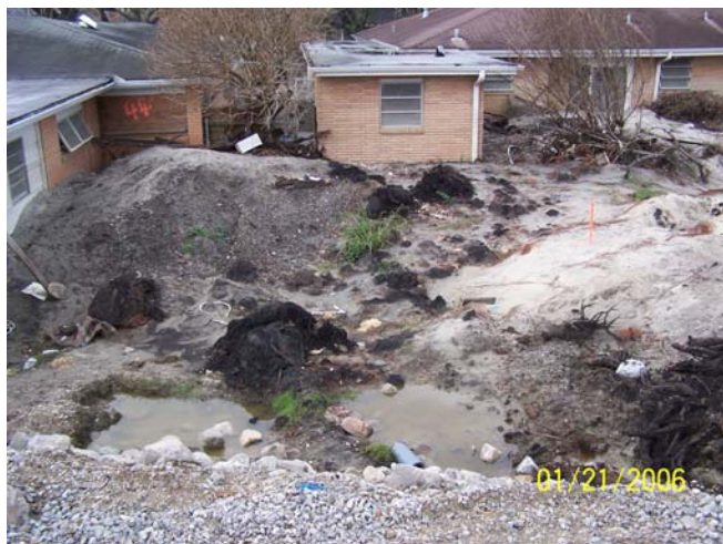
Figure 39. Sand deposits and peat blocks (black) behind homes on Pratt Drive at the North breach of the London Ave. Canal. Note the sand boil on the right. Gray material in the foreground is gravel used in the repair of the breach.
