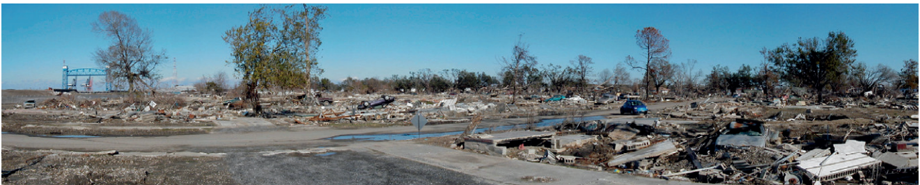
Fig. 5. Near-180° panoramic views in the immediate vicinity of breached levee sites in New Orleans. a. London Avenue Canal, with cranes on the righthand side indicating location of the breach where reparations are ongoing (see Fig. 2c). The open lot in front of the red crane was the location of the home that is in the centre of the panorama and was displaced ~40 m by the flood. Sediment-covered street on the lefthand side is oriented perpendicular to the canal. b. Outwash fan near the London Avenue Canal breach site with cranes on the lefthand side indicating location of the breach. The outwash fan consists predominantly of sands derived from the Pine Island barrier, a sand body that extends up to ~10 m below the surface (Saucier, 1963). Thickness of the fan is in places 1.5 m or more, sufficient to bury cars. Note the largest fan thicknesses in the wake of the remaining homes, separated by channel-like depressions between buildings (a more detailed discussion of this deposit is provided by Nelson & Leclair, 2006). Also note that roofs are nearly intact, testifying to the limited amount of wind damage compared to flood damage. c. Main breach in the Industrial Canal viewed from the Lower 9th Ward. The levee on the lefthand side has been almost completely restored. This area was built up with dense homes that were entirely eradicated. Note the nearly bare terrain near the breach site, giving way to piles of debris and overturned cars to the right. The radius of the area of complete destruction is at least ~400 m. Photos taken in December 2005.
