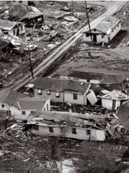
Housing devastation in the Ninth Ward, New Orleans (photo by Paula Burch-Celentano, Tulane University Office of Publications)
